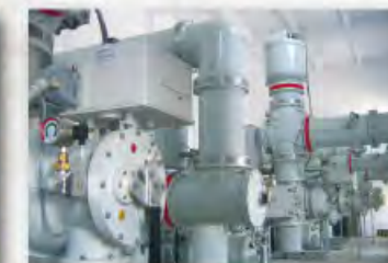
220kV Gangnan Substation Engineering of Xinjiang Electric Power Company
